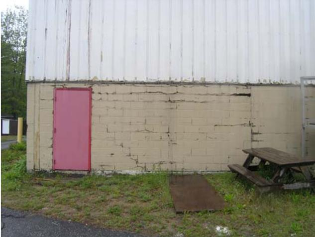
Masonry and Metal Panel Deterioration at Southeast corner
