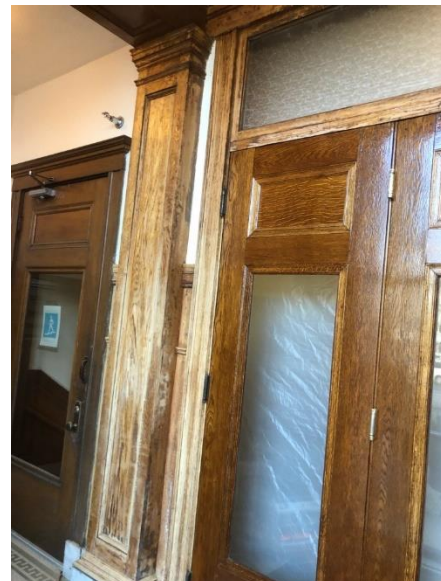
Stripping and Refinishing of Entry-way Door at City Hall
