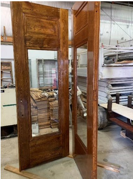
Stripping and Refinishing of Entry-way Door at City Hall
