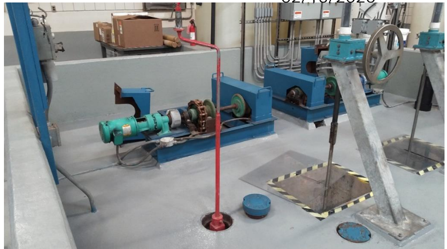
Sedimentation Basic 2 chain Drive repairs in Progress
