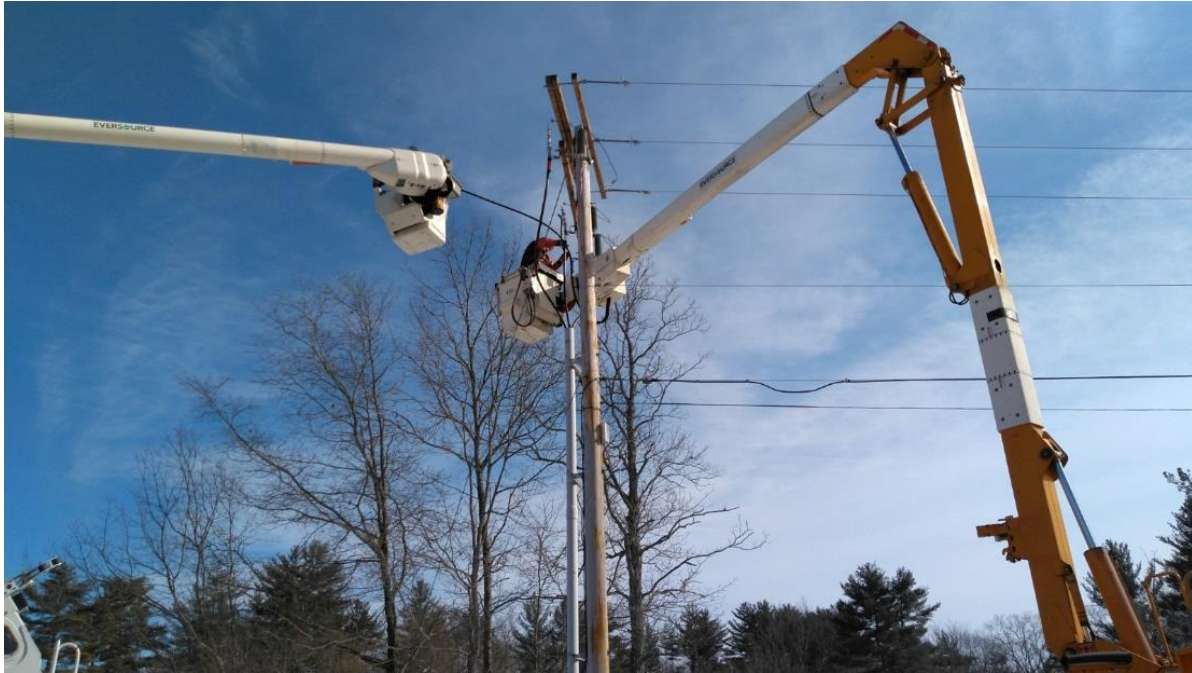
Repairs to power drop at Cocheco Well
