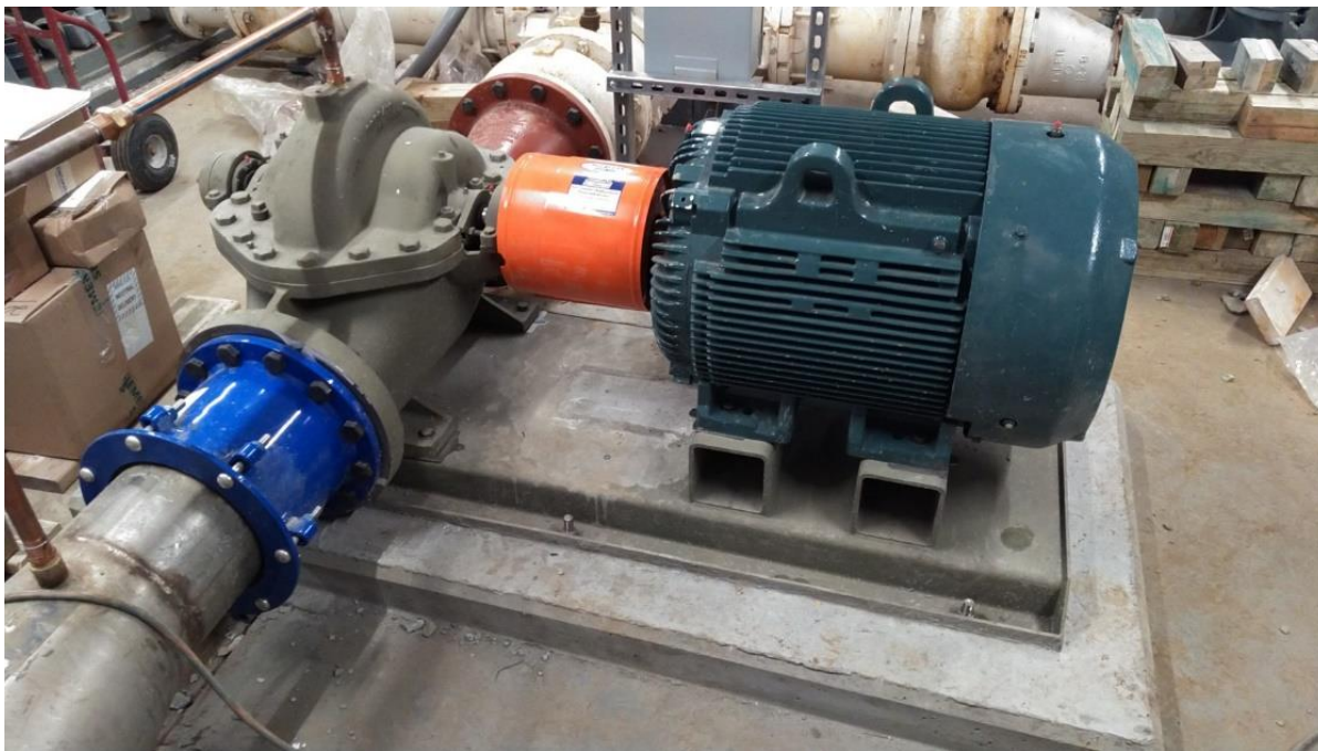
New Raw Water Pump & Motor #2.
