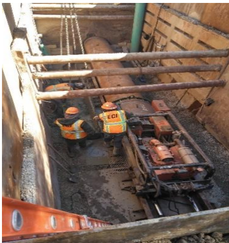
Sleeve for Granite State Business Park/Shaw Drive Water Line
