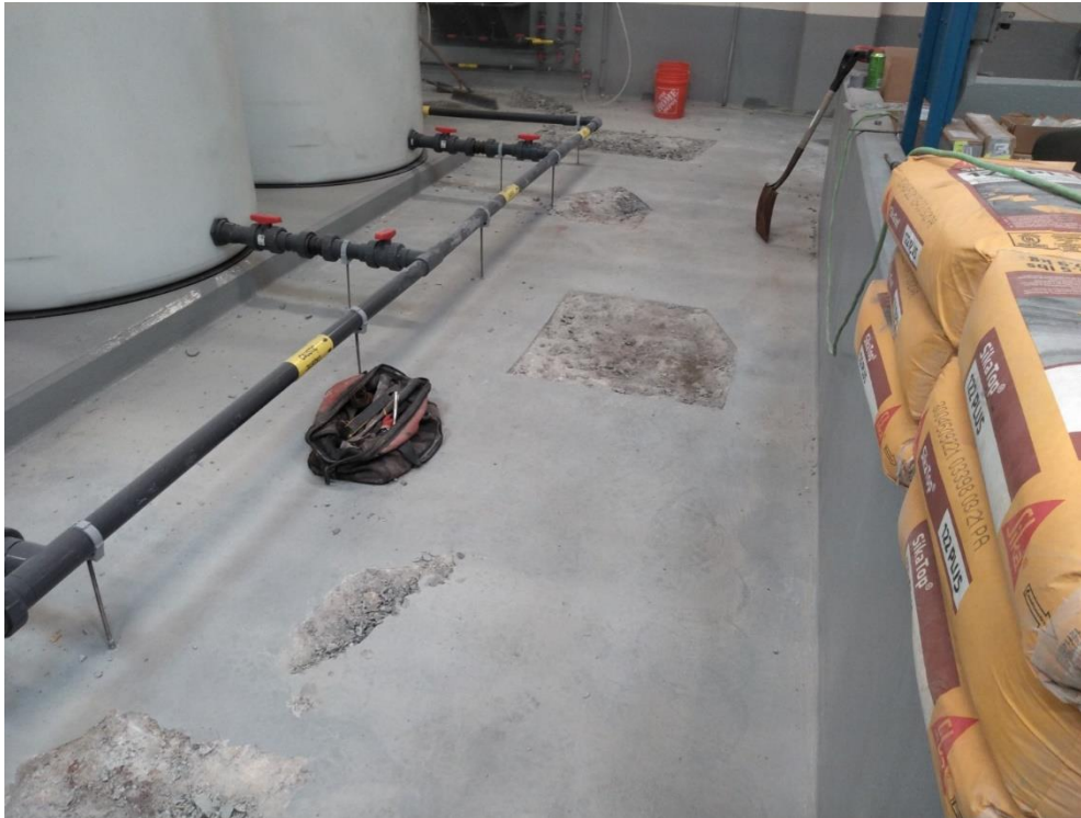
Containment floor repairs underway
