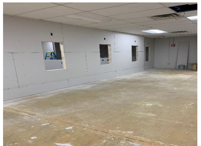
Framing and Sheet Rock the New Tax Office
