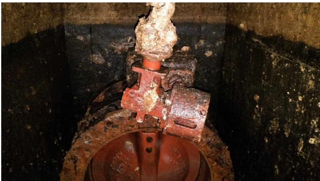
Broken valve actuator
