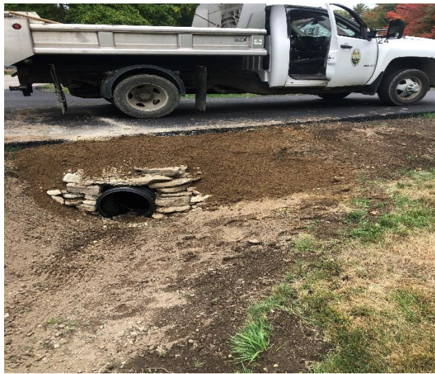
Culvert Repairs 606 Salmon Falls Road
