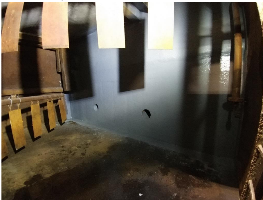
Flocculator Basin Sealed and Cleaned
