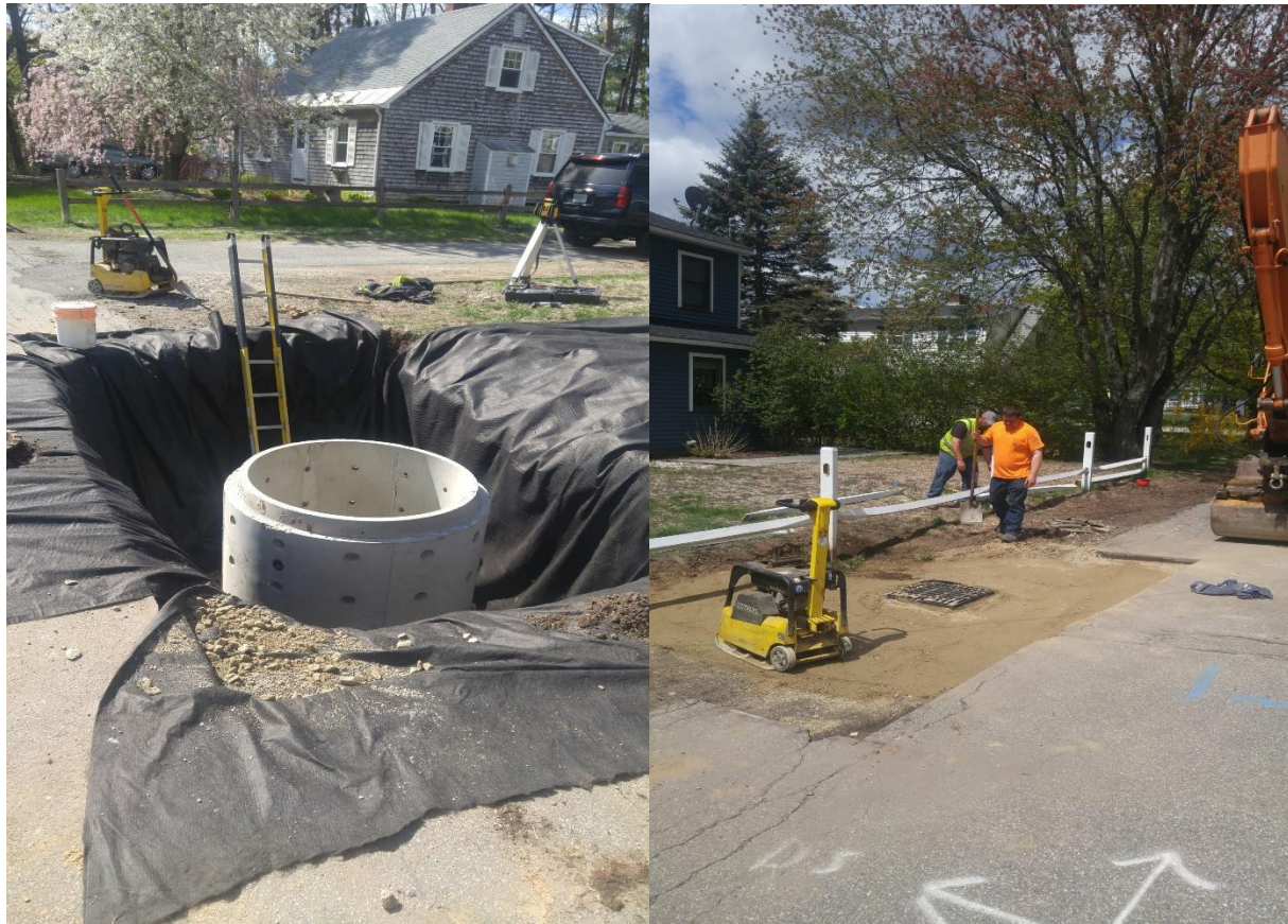
Installation of new dry well on Schley St.
