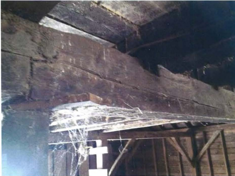
Photo showing cracked beam
