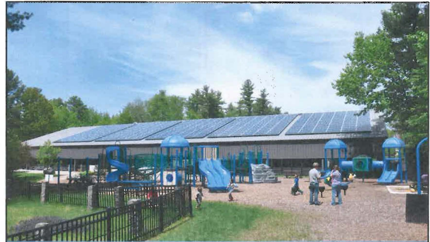
96 kW Grid-Tied Array (120 kW PPA) Churchill Rink, Durham NH
