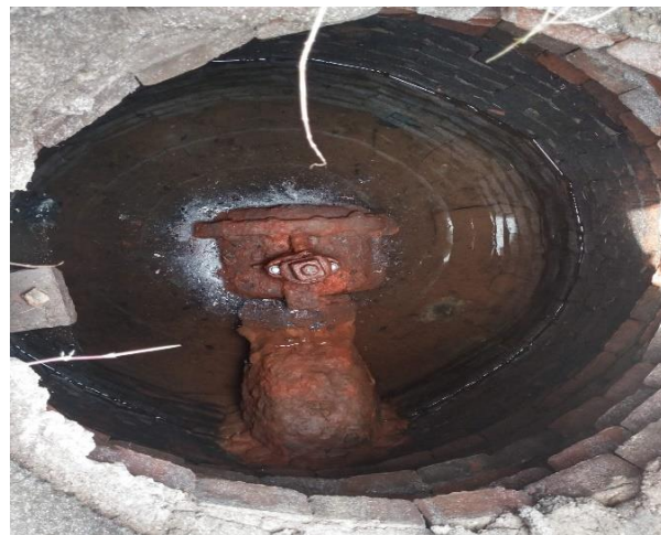
20" gear gate at Washington Street
