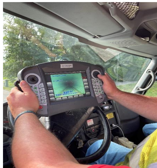
An operator remotely guides a camera thru a sewer main during a mainline inspection
