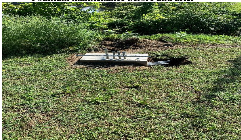
Concrete pad and conduit for electrical service Duval Park
