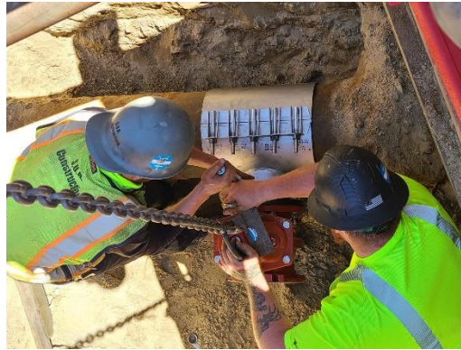
SUR water service tie-over near Sherwin Williams on Old Dover Road
