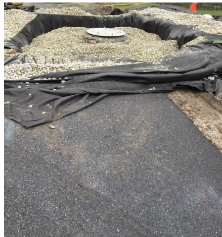
Chestnut Street dry well installation
