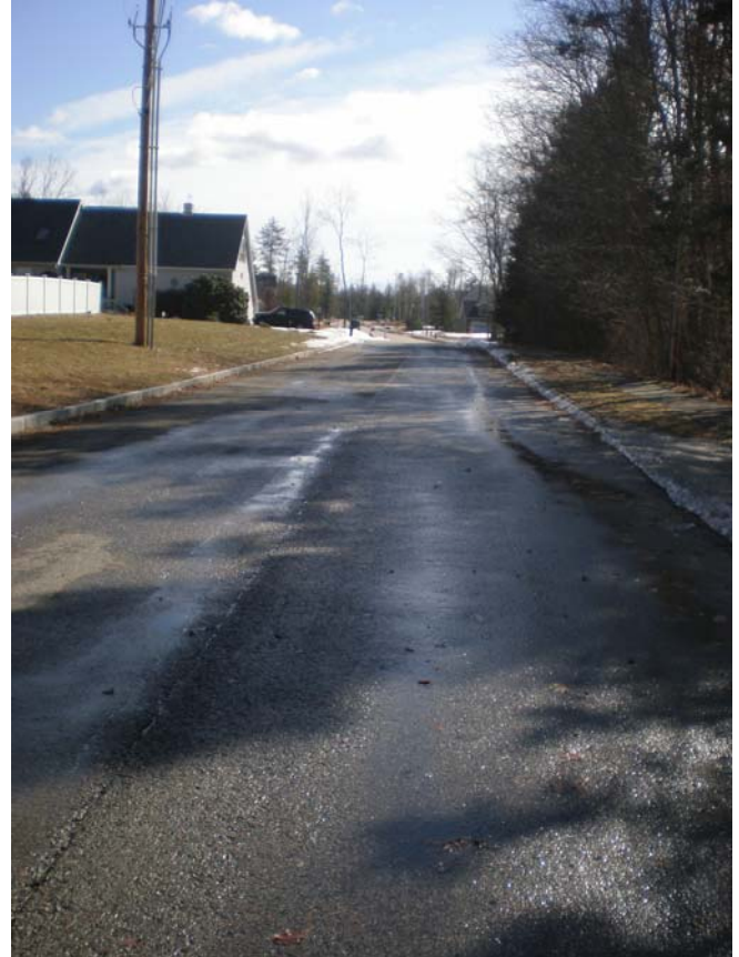
Figs 2-3. Longitudinal crack from Franklin St. in approximately 800 feet to No. 34. The crack indicates inadequate tacking of coats. Crack will at least require saw cutting out. Layering wear course over this will result in reflective cracking in near future. Note the rutting of the road in the wheel tracks. This indicates inadequate base materials and/or compaction thereof.
