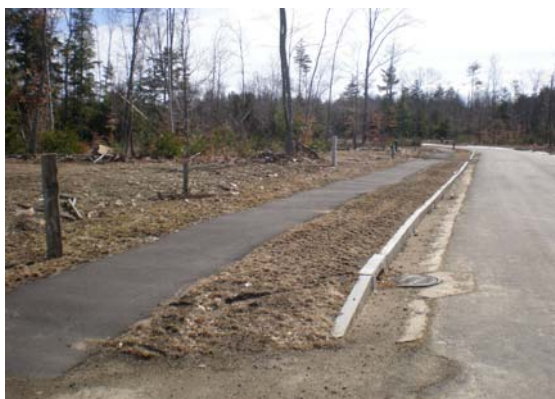
Fig 9. Sidewalk longitudinal and cross slopes are wavy and not ADA compliant. Additional pavement will not solve this problem. Sub-base material is in question.
