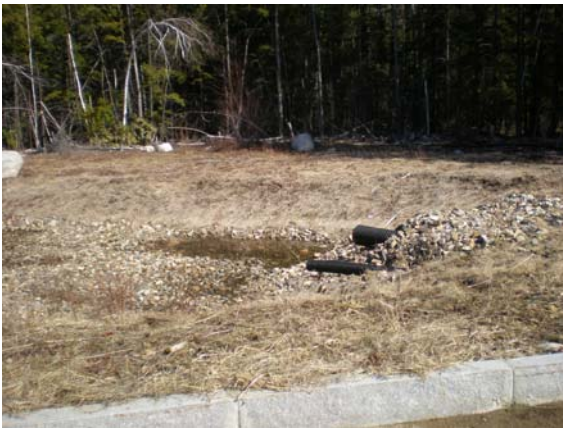
Fig 13. Drainage ponds remain unfinished and apparently modified in configuration from drawings.
