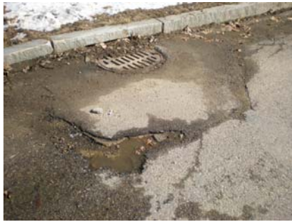
Fig 5. Pavement problems at interfaces with structures.
