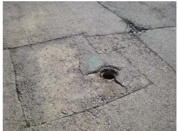
Fig 6. Subsidence near structures indicates inadequate materials and/or compaction thereof. Note missing cover.
