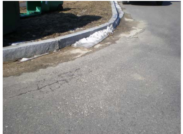
Fig 8. Low shoulder and inadequate compaction results in ponding water.
