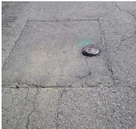
Fig 7. Subsidence near structures indicates inadequate materials and/or compaction thereof. Note missing cover.
