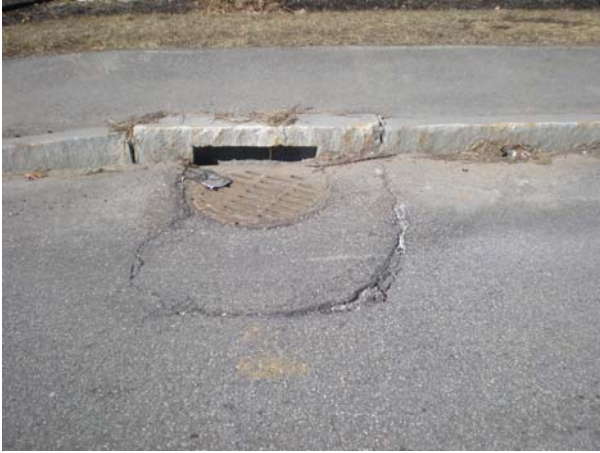
Figs 11-12. Franklin St. drainage structures. Negative drainage due to heaving of structures. Sub-base materials and/or degree of compaction thereof suspect.
