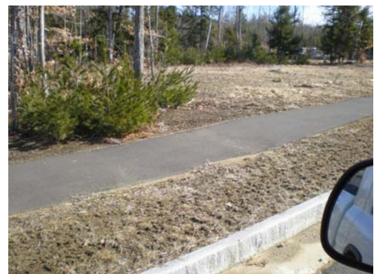
Fig 10. Sidewalk cross-slopes way exceed 2% per code.
