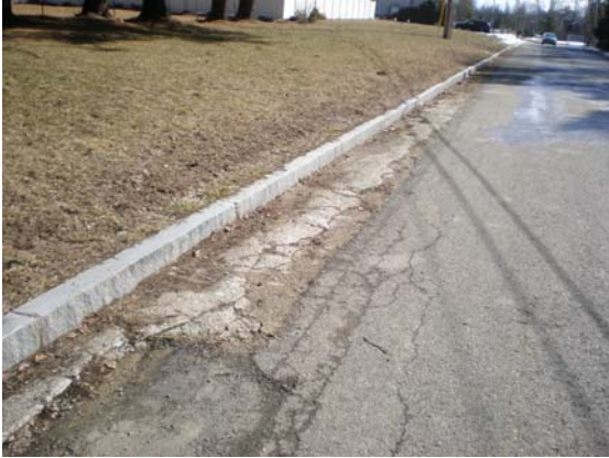
Fig 1. Concrete curb backing in poor condition and rotation of curbing. Cracks are a sign of inadequate compaction of sub materials.
