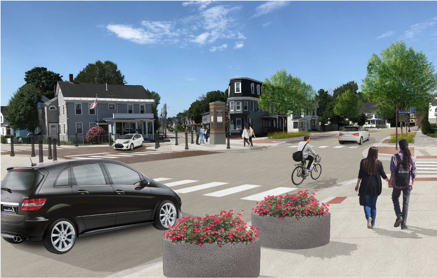
Figure 6: Design concept for North Main Street. The perspective shows two lanes of traffic with shared use lanes, a reconfigured River Street and Pine Street intersection as a pervious paver tabletop, a neighborhood monument, pervious paver parallel parking spaces, stormwater planters, splash guard behind curb, historic lighting, wayfinding signage, and above ground planters.
