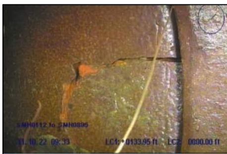
Photo 15: Fracture spiral at STA 1+34
