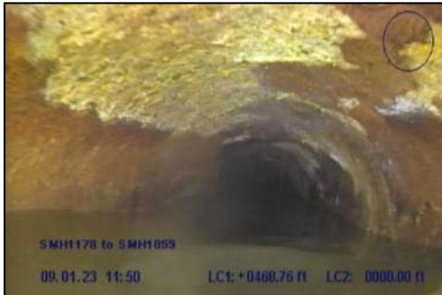
Photo 58: Surface damage missing wall at STA 4+69
