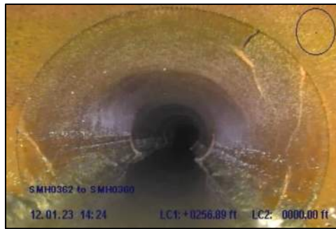
Photo 31: Fracture multiple at STA 2+57
