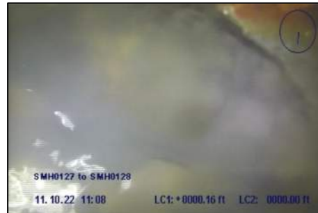
Photo 21: Hole at STA 0+00
