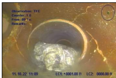
Photo 19: Fracture spiral at STA 0+01
