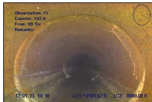
Photo 36: Fracture multiple at STA 1+85
