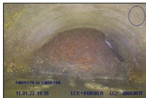
Photo 1: Root Ball in Sewer Segment SP00936 on Eastern Ave at STA 1+90
