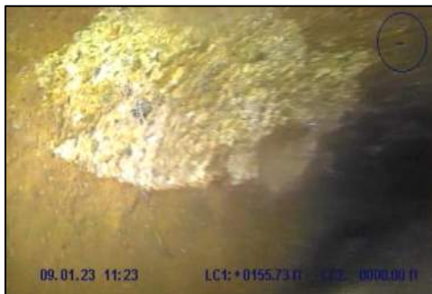
Photo 60: Surface damage missing wall at STA 1+56
