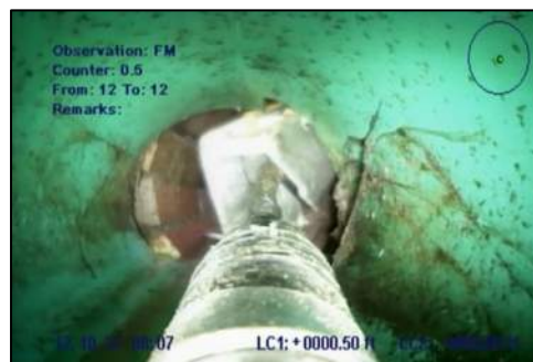
Photo 25: Fracture multiple at STA 0+01
