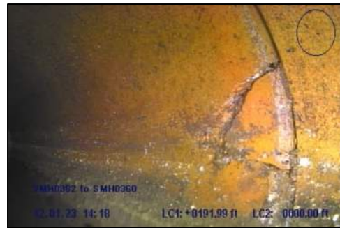
Photo 38: Broken pipe at STA 1+92
