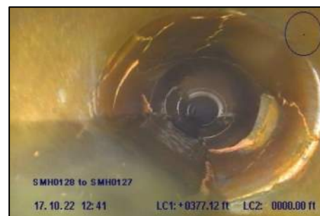
Photo 20: Fracture spiral at STA 3+77
