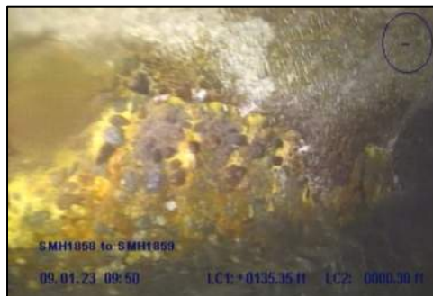
Photo 44: Surface damage missing wall at STA 1+35
