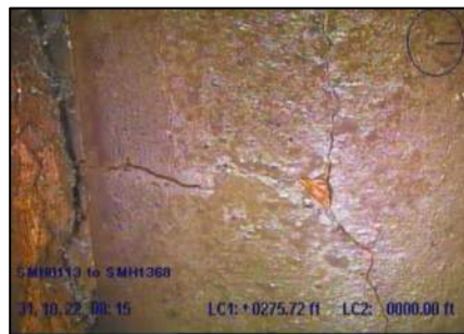
Photo 14: Fracture multiple at STA 2+76
