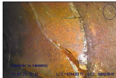
Photo 50: Broken pipe at STA 2+94
