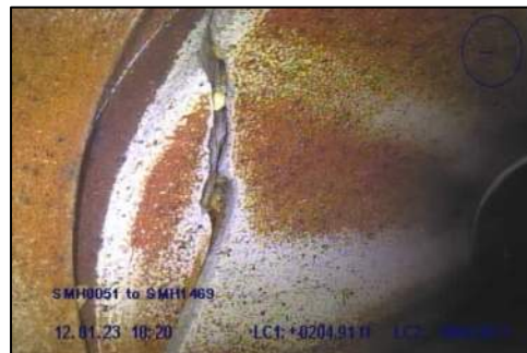
Photo 53: Broken pipe at STA 2+05
