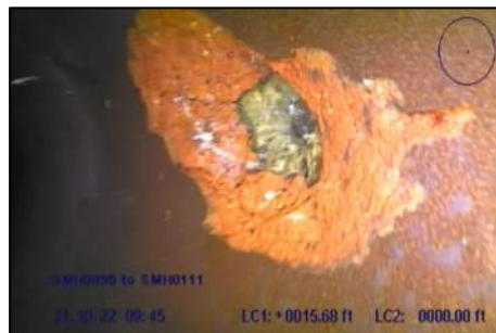
Photo 18: Hole at STA 0+16
