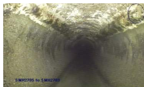
Photo 2: Grease in Sewer Segment SP02126 on River Street
