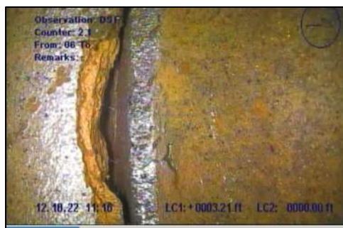
Photo 4: Broken pipe at STA 0+03
