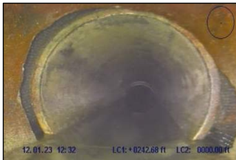
Photo 47: Unknown material under broken pipe at STA 2+44
