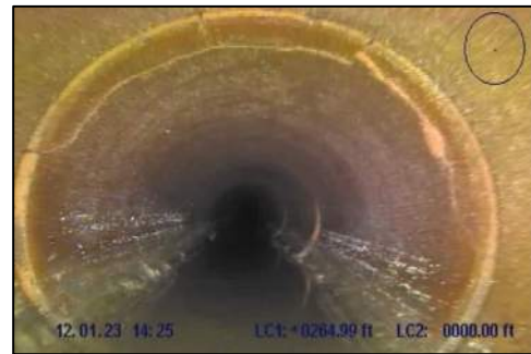
Photo 32: Fracture spiral at STA 2+64
