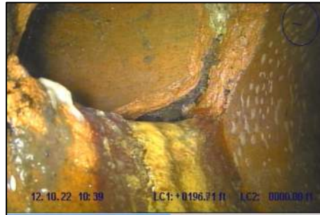
Photo 17: Hole void visible at STA 1+97
