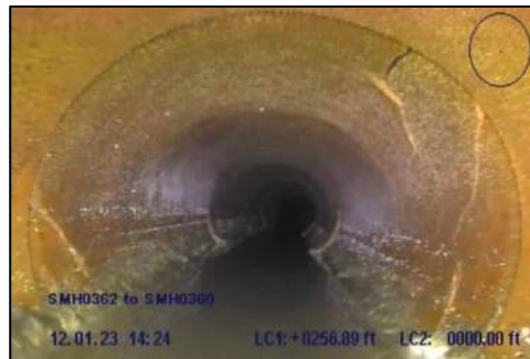
Photo 33: Fracture multiple at STA 2+90
