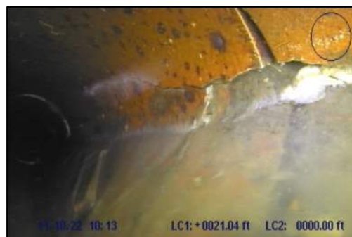
Photo 23: Hole at STA 0+21
