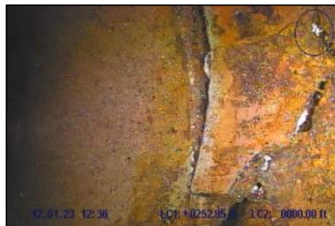
Photo 49: Broken pipe at STA 2+53
