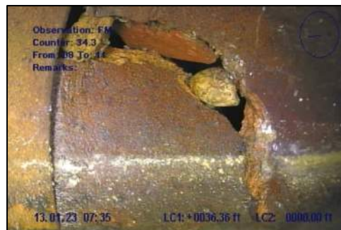
Photo 40: Hole void visible at STA 0+36
