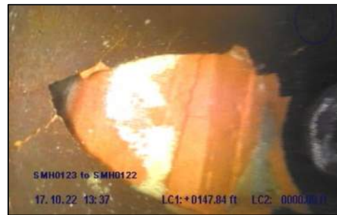
Photo 10: Hole at STA 1+48
