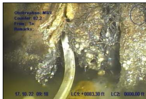
Photo 6: Plastic in joint at STA 0+83
