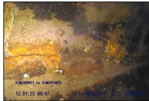
Photo 52: Fracture multiple at STA 0+25
