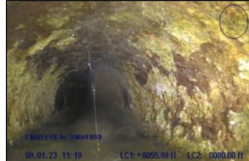
Photo 59: Surface damage missing wall at STA 0+55
