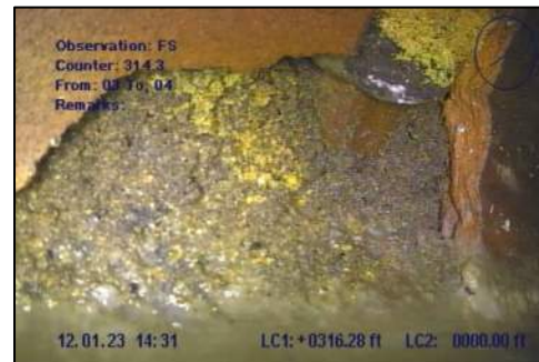
Photo 28: Hole soil visible at STA 3+16
