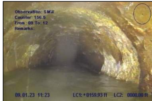
Photo 61: Surface damage missing wall at STA 1+60
