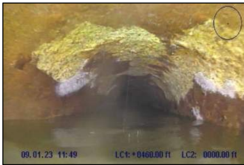
Photo 56: Surface damage missing wall at STA 4+61
