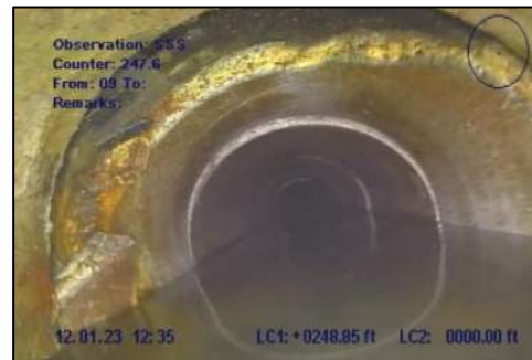
Photo 48: Unknown material under broken pipe at STA 2+50
