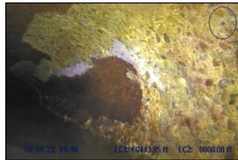
Photo 57: Surface damage missing wall at STA 4+44
