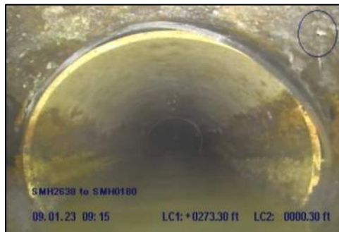
Photo 43: Joint connection lining defect at STA 2+75
