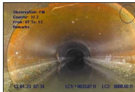
Photo 39: Fracture multiple at STA 0+34
