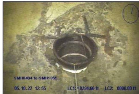
Photo 26: Surface damage at STA 2+95
