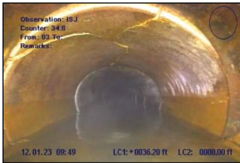
Photo 51: Fracture multiple at STA 0+37
