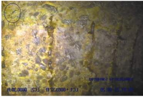
Photo 41: Surface damage reinforcement visible at STA 0+03
