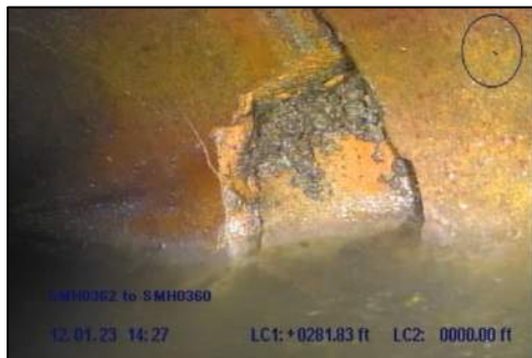
Photo 27: Hole at STA 2+82
