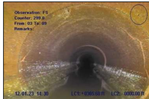
Photo 34: Fracture spiral at STA 3+06
