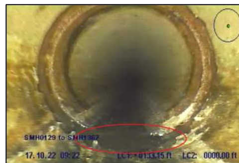
Photo 8: Hole at STA 1+34
