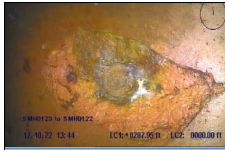
Photo 11: Surface damage missing wall at STA 2+88
