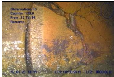
Photo 37: Broken pipe at STA 1+31
