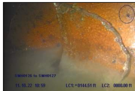
Photo 22: Fracture spiral at STA 1+45
