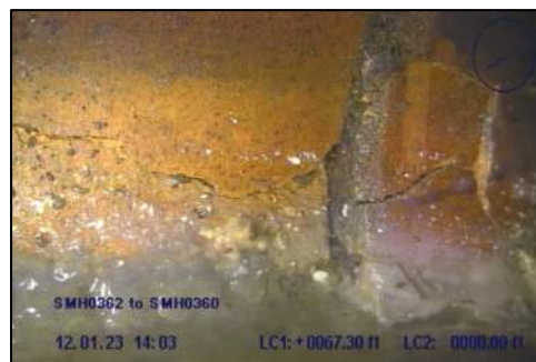
Photo 29: Fracture multiple at STA 0+67
