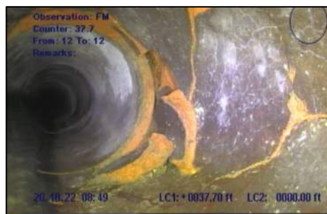
Photo 12: Fracture multiple at STA 0+38
