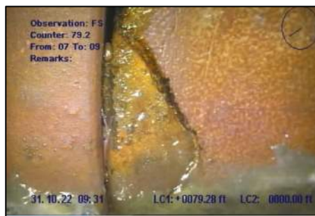
Photo 16: Fracture spiral at STA 0+79
