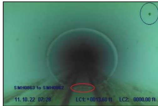
Photo 24: Hole at STA 0+14
