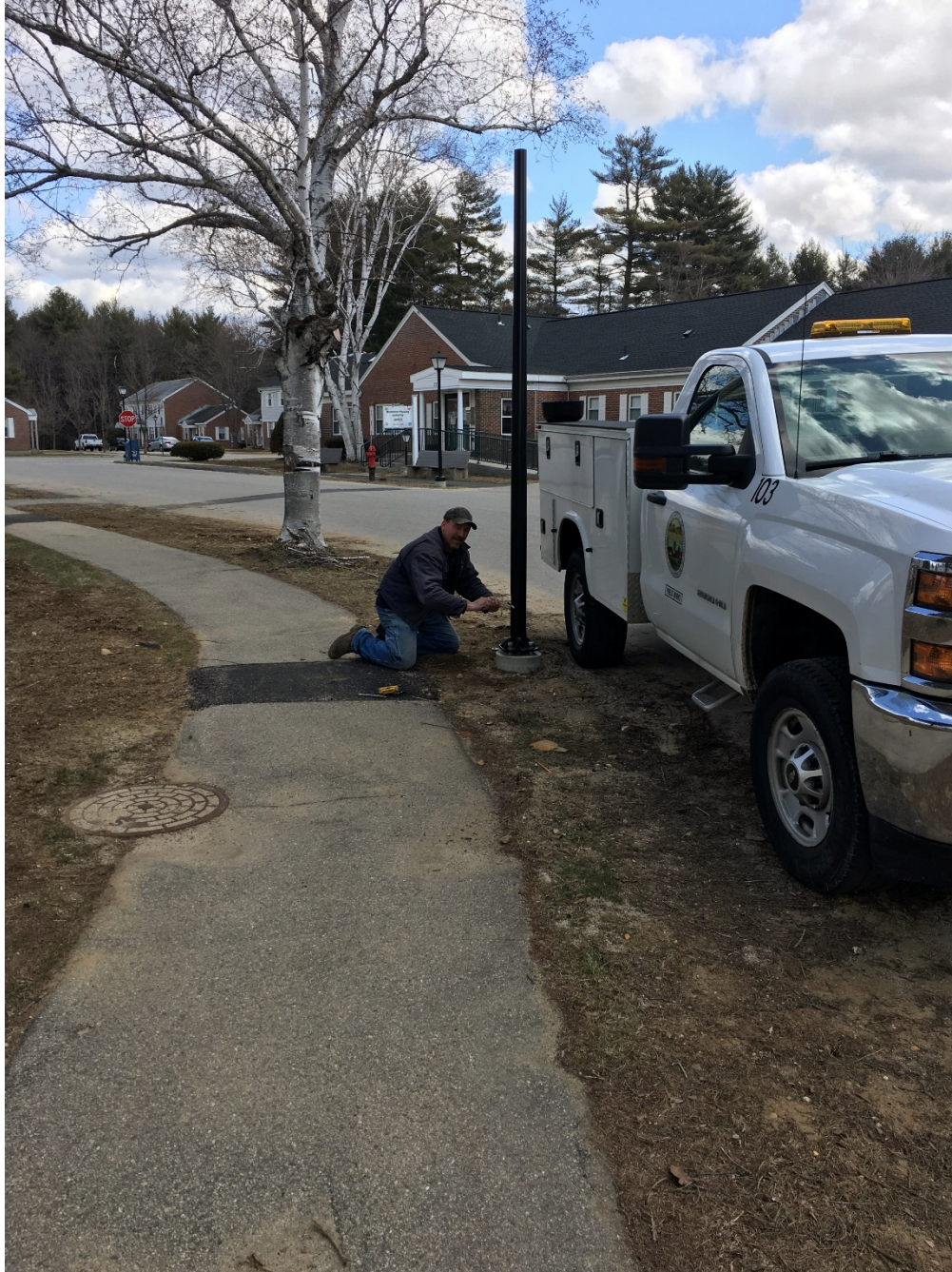
Replacing damaged light pole
