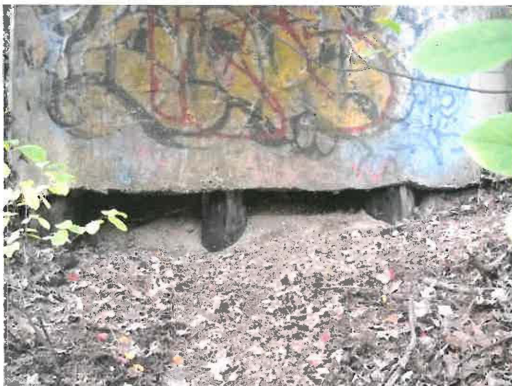
Abutment 2 Undermining
