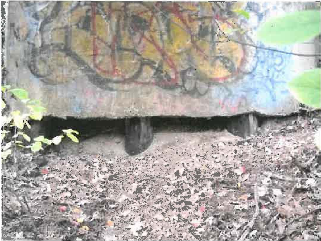
Abutment 2 Undermining
