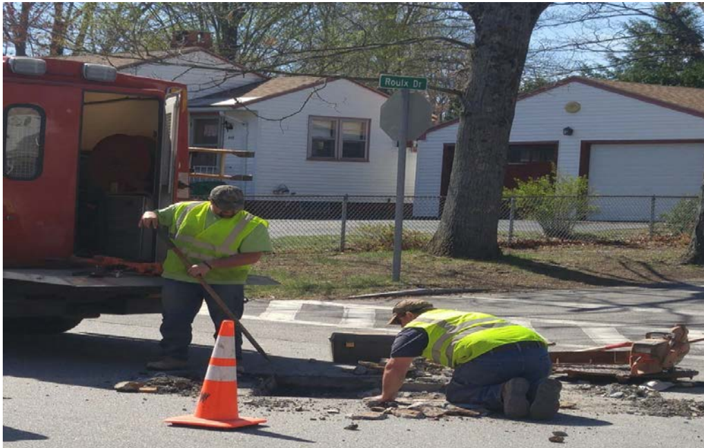
George Steele & Bill Prentice resetting a fallen manhole in the road.
