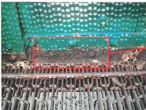
Span 3 Interior Bottom Flange Vertical Leg
