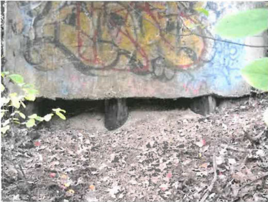
Abutment 2 Undermining
