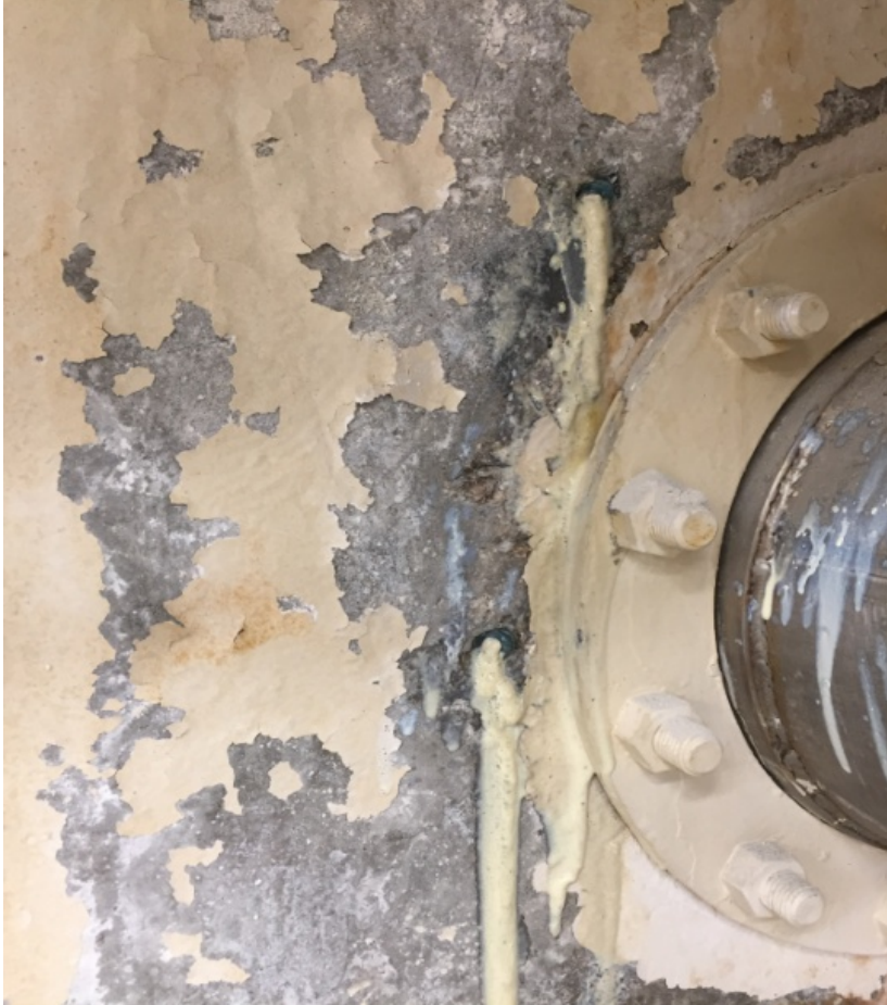
Pipe gallery in process of leak sealing
