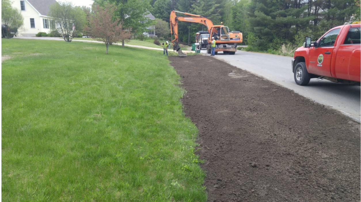
Filling & loaming Tessier Drive ditchline
