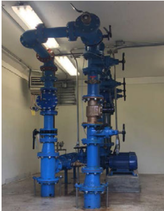
Industrial Way Pump Station Surge Bypass Installation
