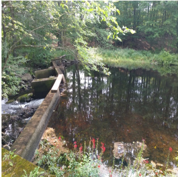
Diversion Dam supplying over 2cfs to the Isinglass
