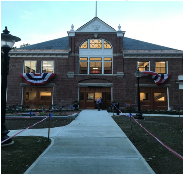
City Hall Annex
