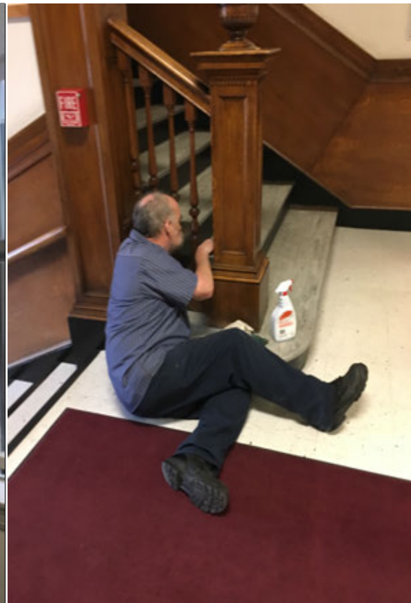
Detailed cleaning of the woodwork at City Hall
