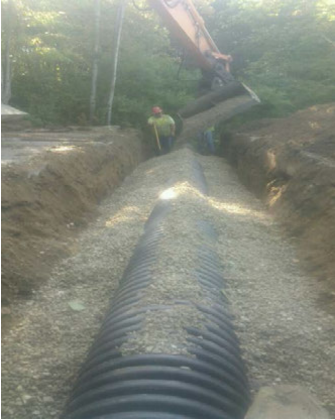
Left Photo- Four Rod Road Drainage Repair
