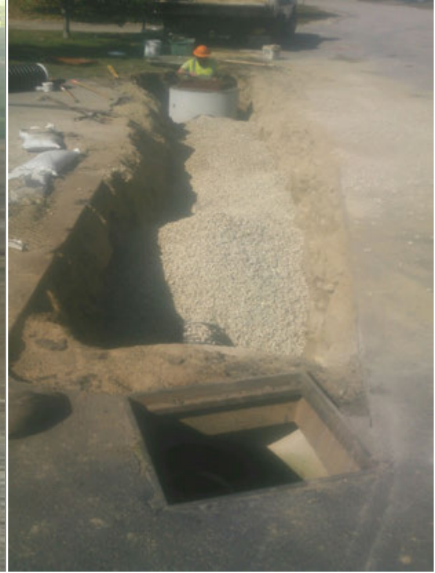
Right- Violet Court Catch Basin Installation
