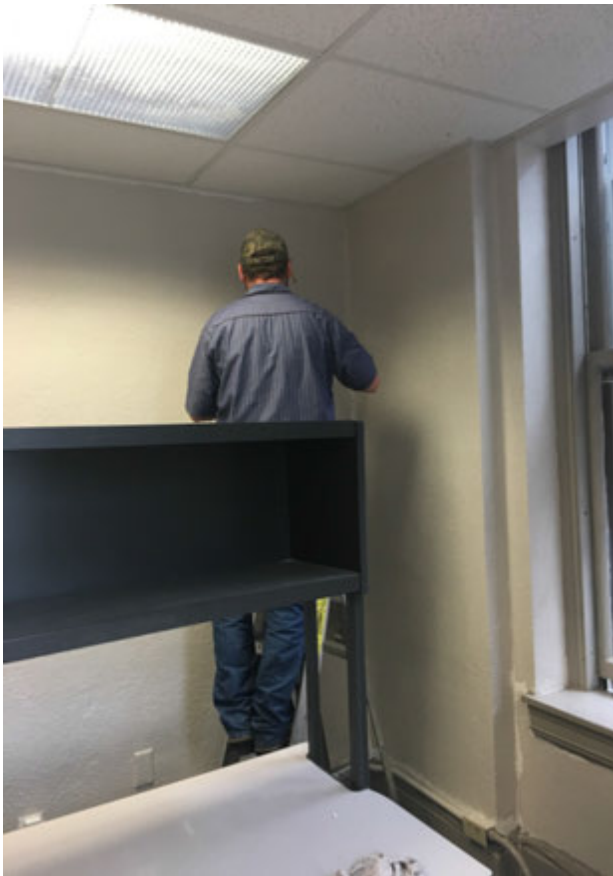
Prepping Walls in Old Codes Office
