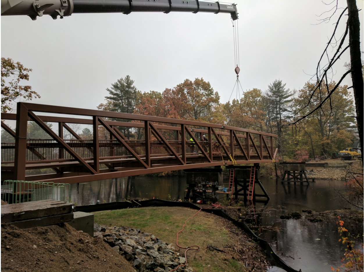
Placement of the new Dewey St. Bridge
