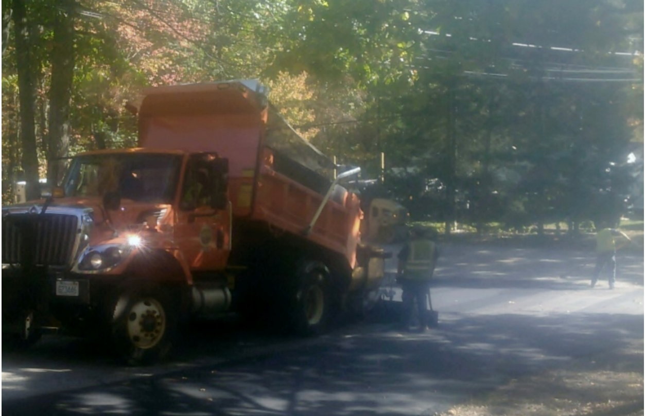
Paving on Pine Knoll Drive
