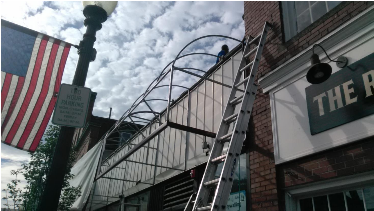
Removal of 1970s/1980s awning from the building
