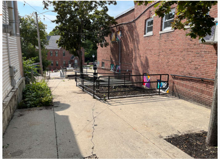
Closer View from North Main looking toward Wyndotte
