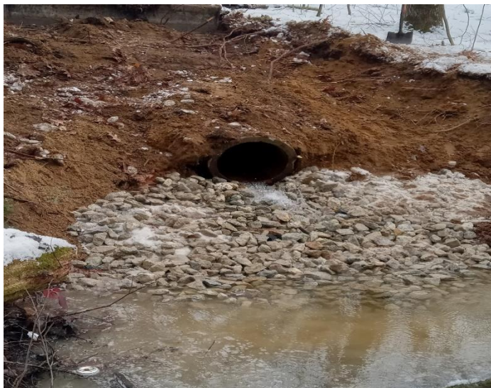
Blackwater Road Culvert
