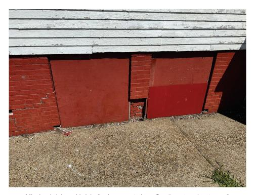
Missing brick and brick displacement along Southeast perimeter wall
