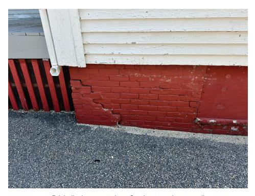
Brick displacement along Southeast perimeter wall
