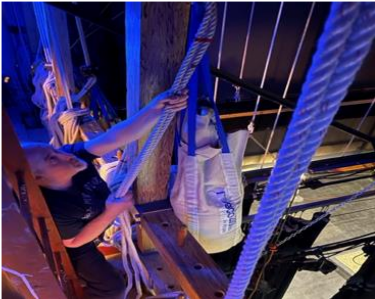
The “Fly Line” above stage left. Nylon lines securing lighting batons with sandbags for counter weight
