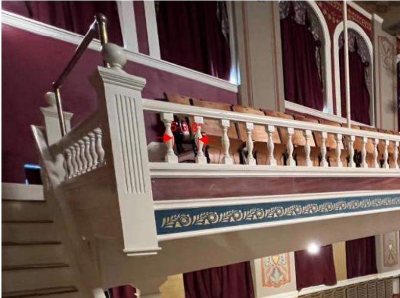
Figure 14 – Balcony Railing Balusters
