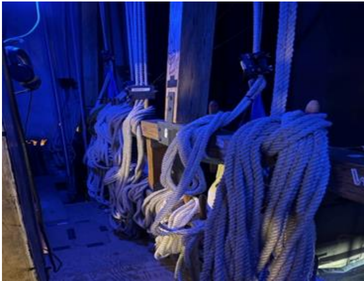
The “Fly Line” above stage left. Nylon lines securing lighting batons with sandbags for counter weight
