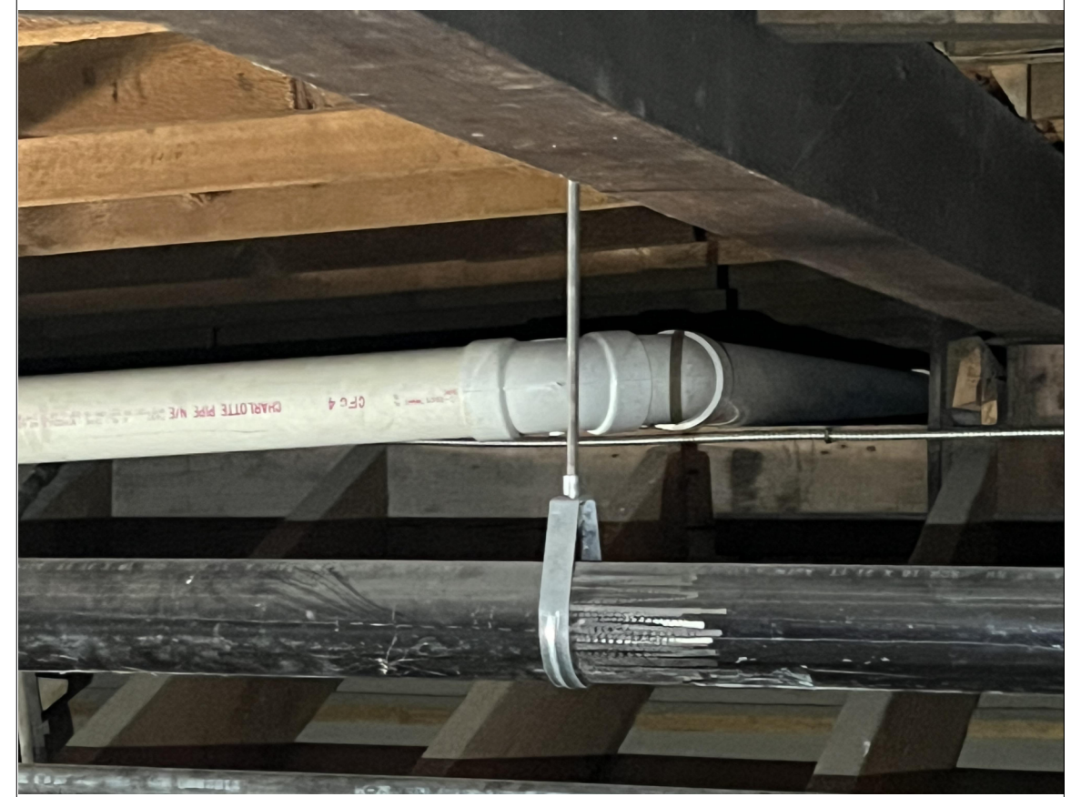
PICTURE 2 - EXISTING 4" PVC ROOF DRAIN
