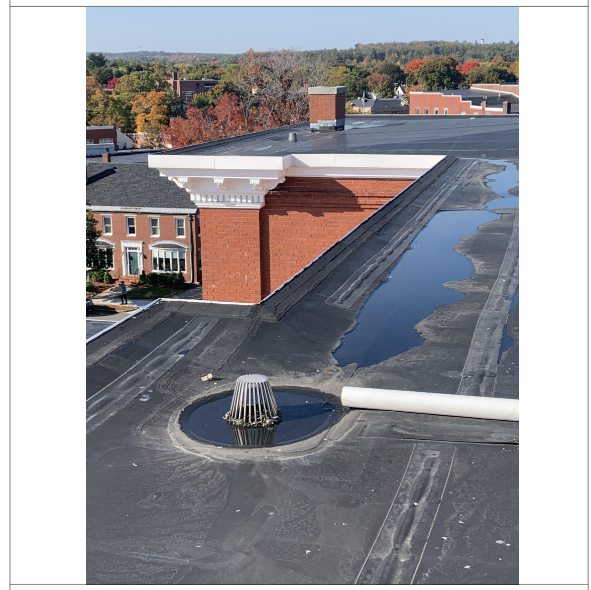
PICTURE 2 - EXISTING ROOF DRAIN RD-3E
