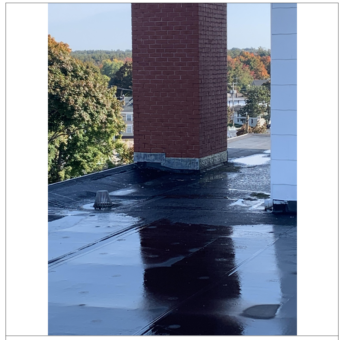
PICTURE 1 - EXISTING ROOF DRAIN RD-2E
