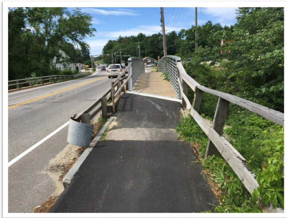
North Approach Looking South
