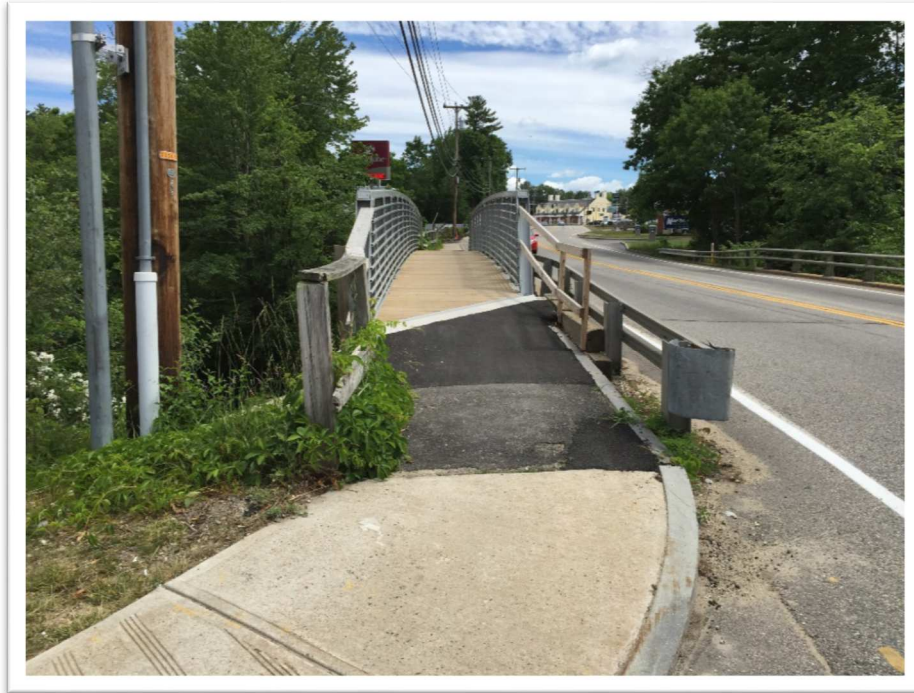
South Approach Looking North
